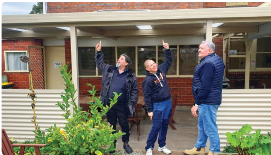
Right: Grant recipient, Lazarus House who support the homeless community, revealing the new roof over their outdoor seating area, allowing people to share meals and social connection sheltered from the weather.
